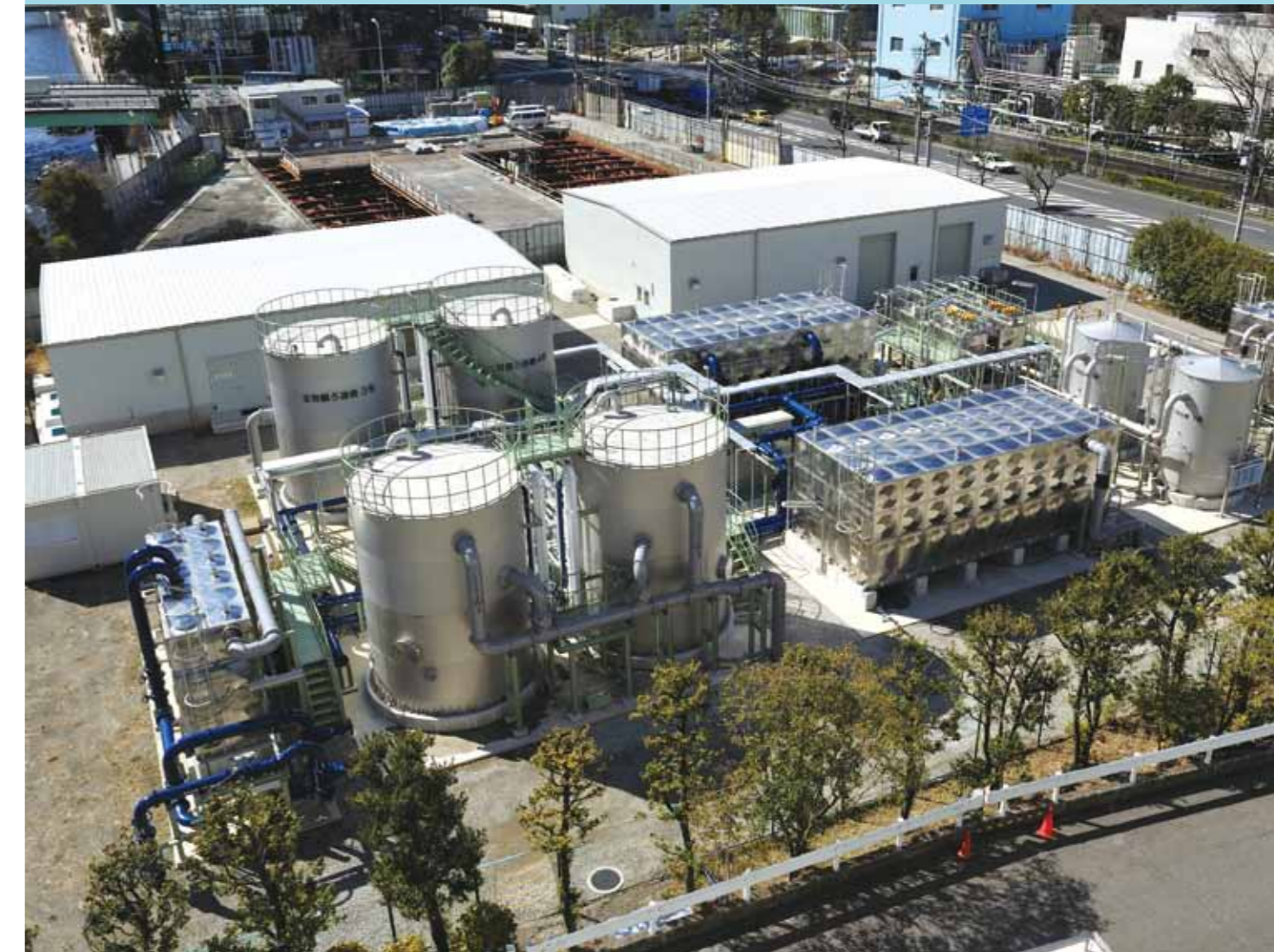
Shibaura Water Reclamation Center
